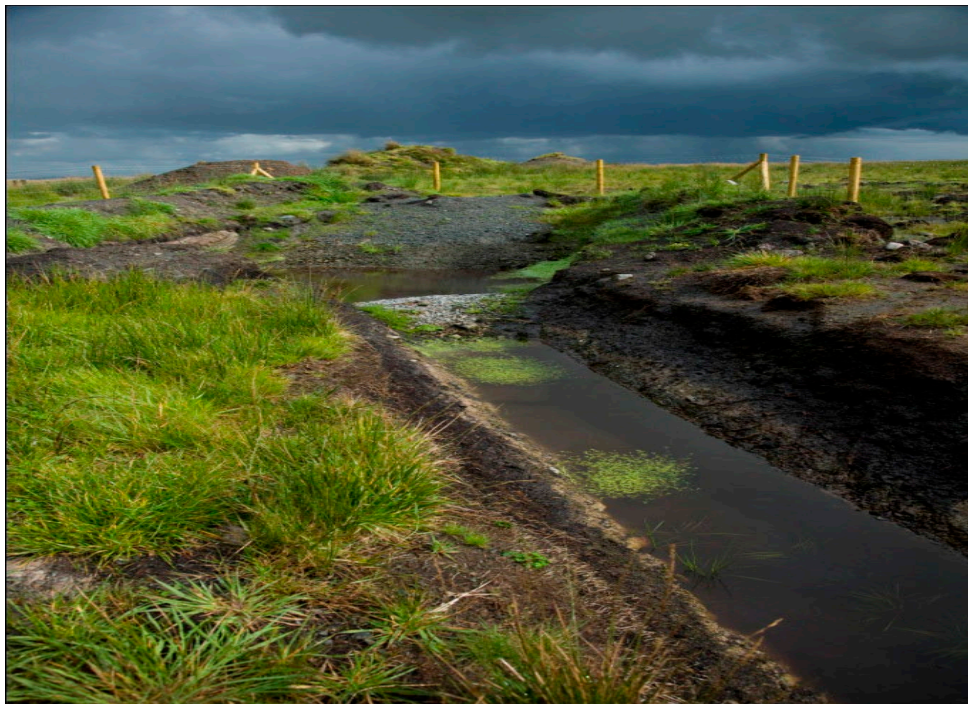
Image 2-4: Swale draining to Settlement Pond
