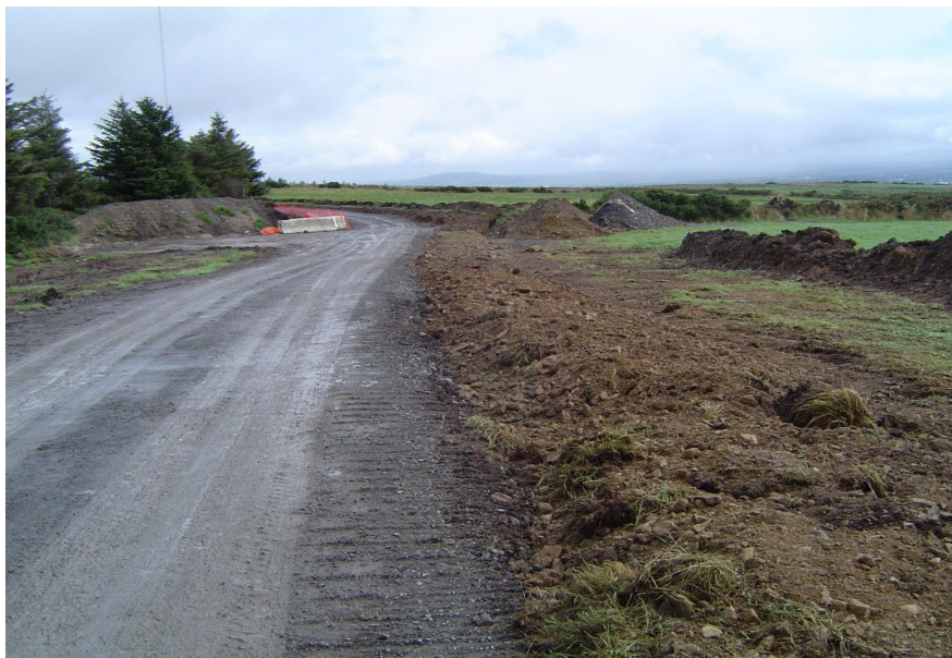
Image 4-3: Backfill over Cable Trench
