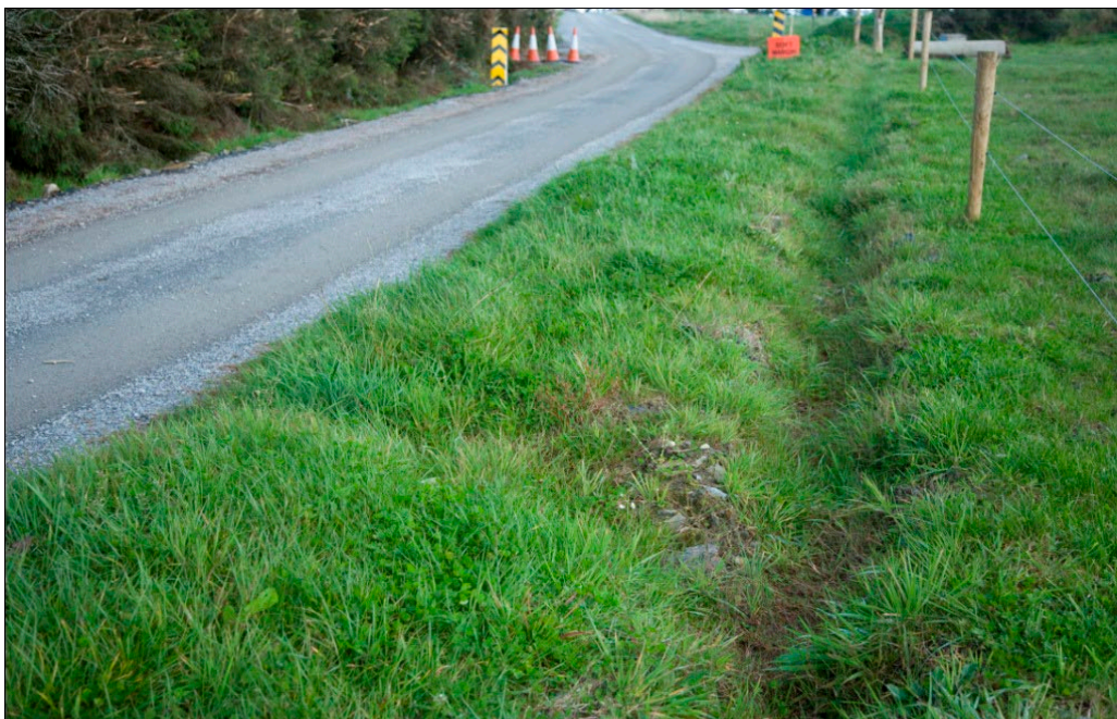
Image 2-2: Grassed swale along access track
