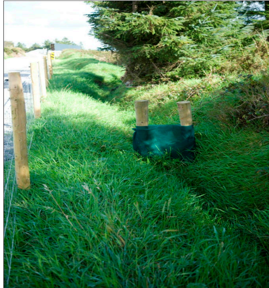
Image 4-1: Silt trap across grassed swale
